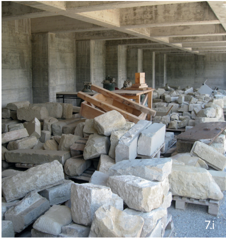
Accumoli, Santa Maria della Misericordia Church, type A debris management: storage of recovered stone and wooden elements in a covered area near the church 7i © Maria Agostiano 7i © Alessandro Betori
