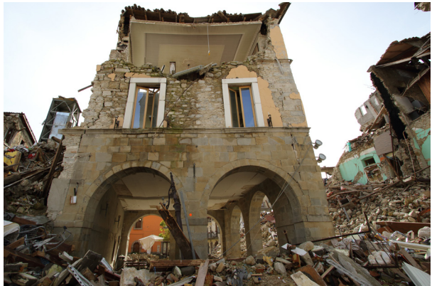
4. Amatrice, historic centre, type B debris © Maria Agostiano
