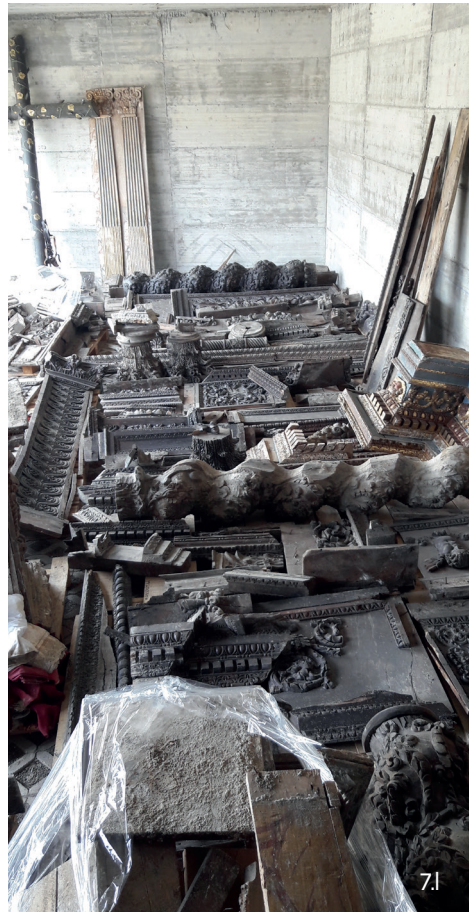
Accumoli, Santa Maria della Misericordia Church, type A debris management: storage of recovered stone and wooden elements in a covered area near the church 7i © Maria Agostiano 7i © Alessandro Betori
